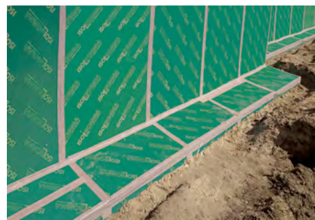
Residential complex foundation, Poland.
